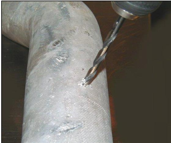
Figure 6 Drill using a 1/4 inch bit.
