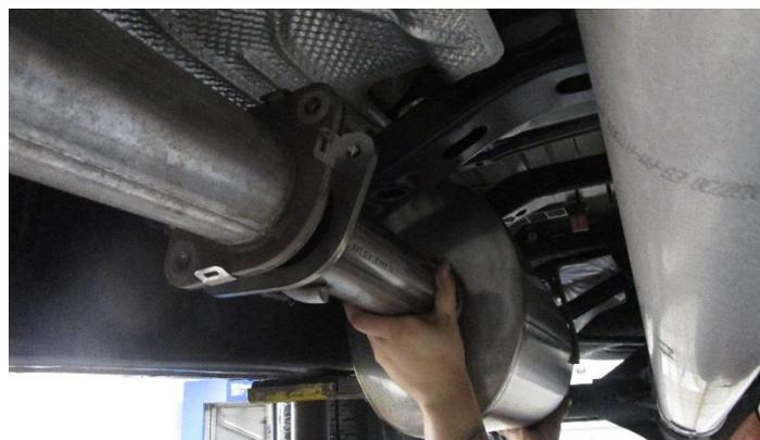
**2.** Line up muffer as shown in the picture. Align the flange to the mating flange of the mid pipe.
