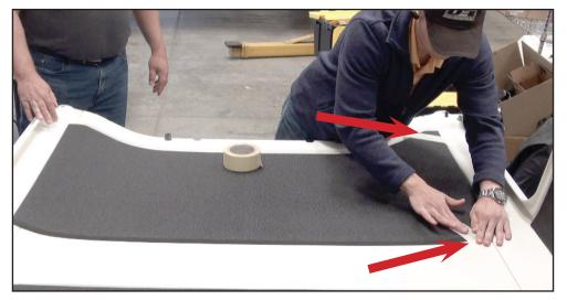
11.) Lay correct piece in removable top. Once again use painters tape to temporarily hold pice in place. Fig 13
