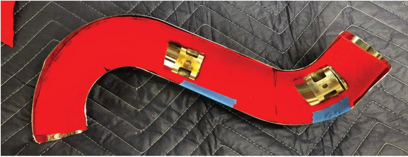
12. You now have a pattern to use to mark and cut the insulation and aluminum. (Fig. 11)
